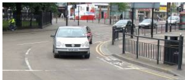
Stratford gyratory ; lane wrong side of railings
