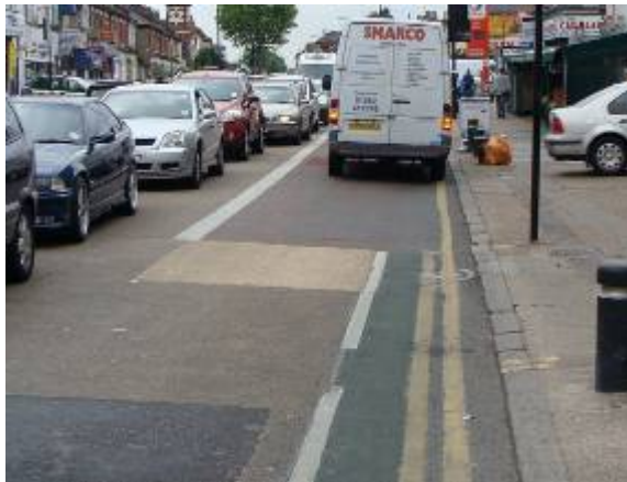
A118 Newham: narrow cycle lane; bus lane blocked
